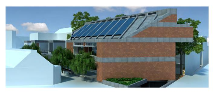
aid in natural ventilation. The project has been monitored continuously during construction and will continue to be monitored after occupation. In its attempt to combine state-of-the-art technology with passive technologies rooted in the tradition of the area, architect BV Doshi sees this architecture sitting at the edge of new trends of thought, suitable not only to India but also to the future, in and outside the country. The building builds on past knowledge but looks toward the future.
